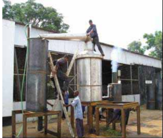
Assembling the still for lemon grass distillation
