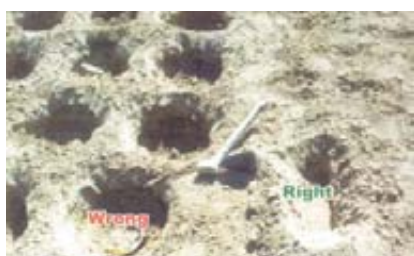
Picture 2. Potholing on the left the holes are wrong while the pothole on the right is the way it should be
